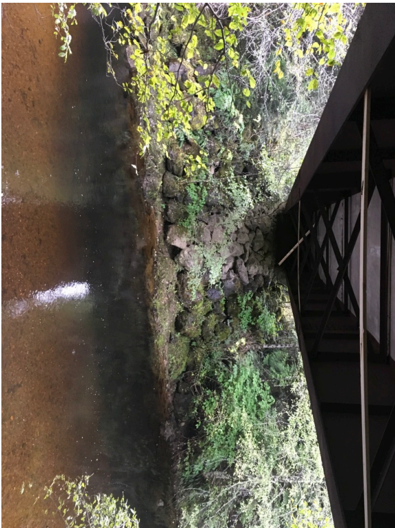
Left Bank Abutment when facing downstream
